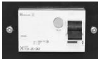
32A D-Curve Switch 30 mA differential
